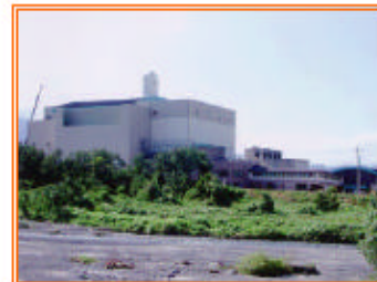
For: Kyohoku Regional Administrative Association 80 ton/day 2 trains Start Const. 2001 *Completed March 2003
