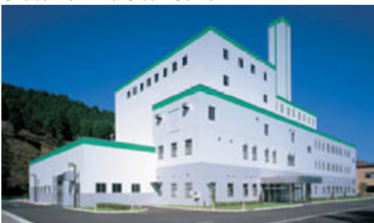
Environmental Sanitation Center, Waste Treatment Facility, Kazuno City
