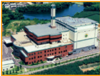
For: Yame Seibu Regional Administrative Association 110 ton/day 2 trains Start Const. 1997 *Completed March 2000
