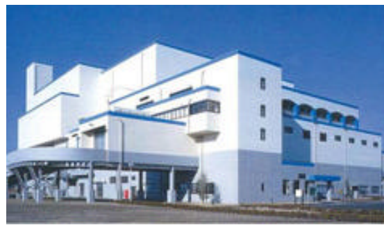
Ishinomaki Area Clean Center
