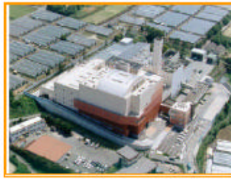
For: Toyohashi City 200 ton/day 2 trains Start Const. 1998 *Completed March 2002
