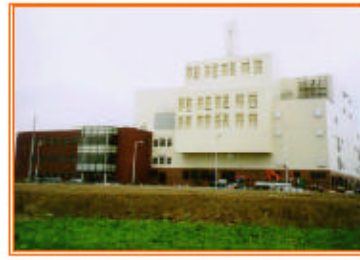
For: Ebetsu City 70 ton/day 2 trains Start Const. 2000 *Completed Nov. 2002
