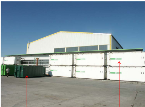
Newer container design attached to the process Bio-drying container Fig. 22 – Impianto di Rügen (Germania) [1]
